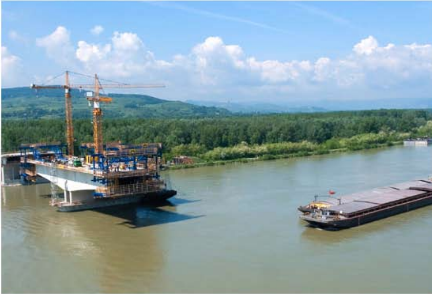
Construction of Traismauer Bridge over the Danube.
