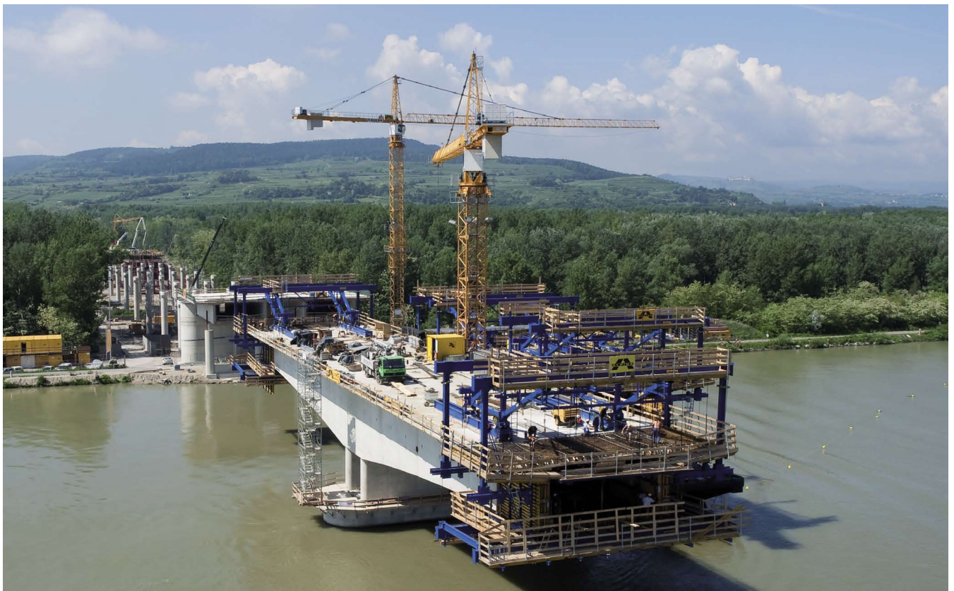
Construction of Trismauer Bridge over the Danube.
